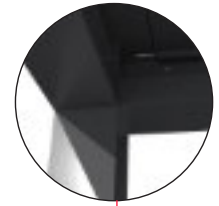
NO VISIBLE SCREWS CONNECTING THE GUTTER WITH THE BASE OF THE PERGOLA
